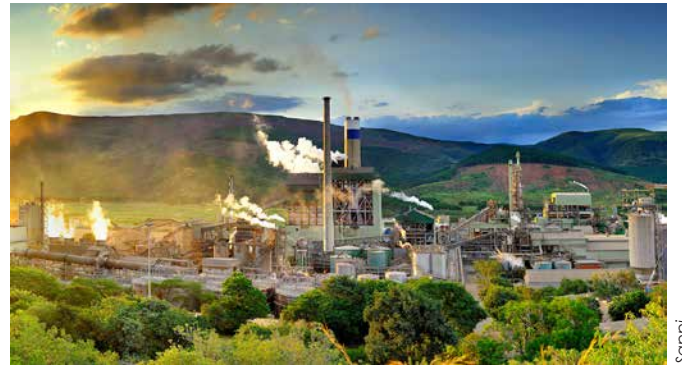
South Africa's first biomass power plant to be constructed under the Renewable Energy Independent Power Producer Procurement Programme (REIPPPP) will soon become operational at Sappi's Ngodwana Mill in Mpumalanga.
