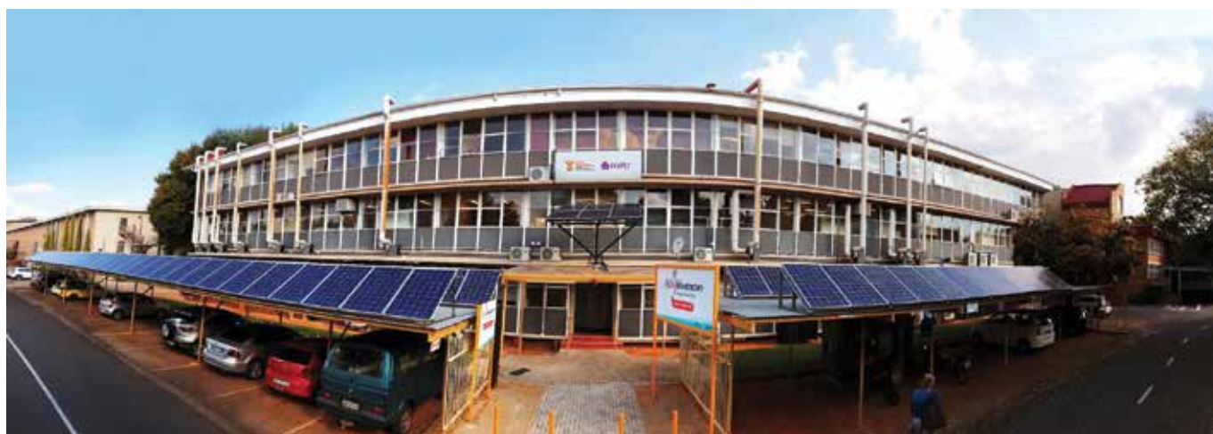
HySA Infrastructure's solar-to-hydrogen facility on the NWU Potchefstroom campus relies on a 55 kW photovoltaic (PV) installation and an electrolytic hydrogen-generation system.
