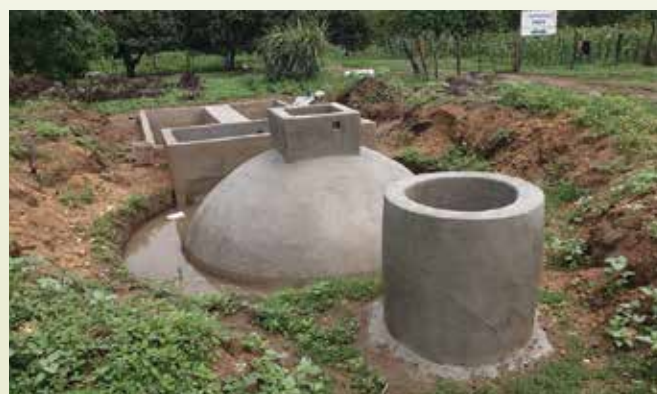
A rural household's newly completed digester, constructed as part of the Waste-to-Energy South Africa Project, which is supported by the United Nations Industrial Development Organisation (UNIDO) and the Global Environment Facility (GEF).
