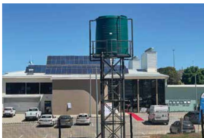
The Cofimvaba Science Centre in the Eastern Cape, officially opened on 6 October 2021, has an electrolytic hydrogen-generation system coupled to a 35 kW solar PV system and a 5 kW hydrogen fuel cell installed by HySA Infrastructure.
