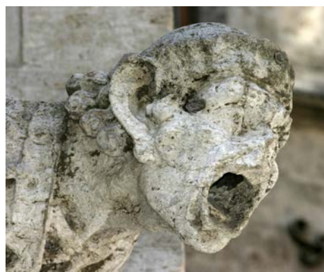
Acid rain dissolves the calcite in marble and limestone, causing damage to buildings and statues.
