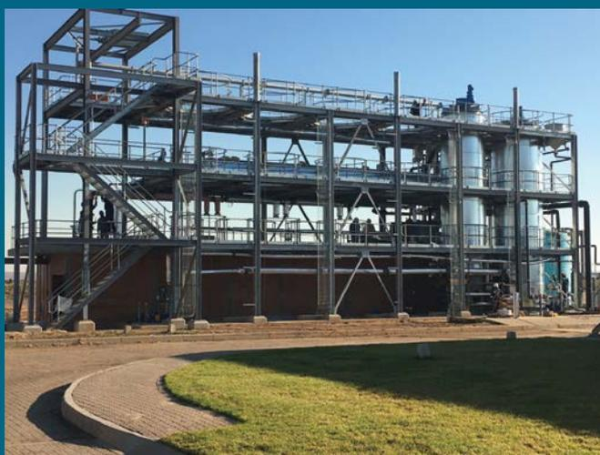
The eutectic freeze crystallisation (EFC) unit designed and built by Prentec at the Tweefontein Colliery in Mpumalanga, based on research done at UCT's chemical engineering department. Much of the research was funded by the Water Research Commission.
