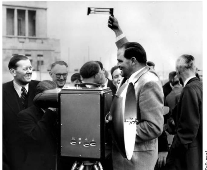
Trevor Wadley using a whirling hygrometer to measure humidity while demonstrating his tellurometer in England in 1957.
