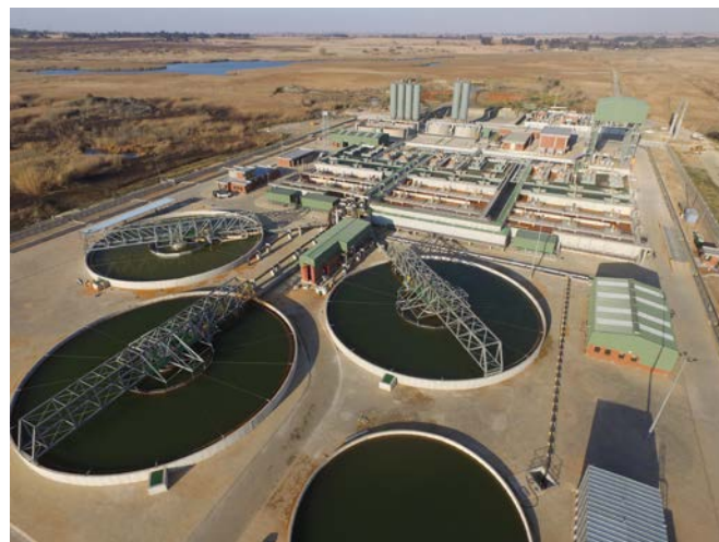
The Eastern Basin AMD treatment plant, designed by AECOM for the Trans Caledon Tunnel Authority (TCTA), is one of the largest high-density sludge (HDS) plants in the world, with a maximum treatment capacity of 110 ML/d.
