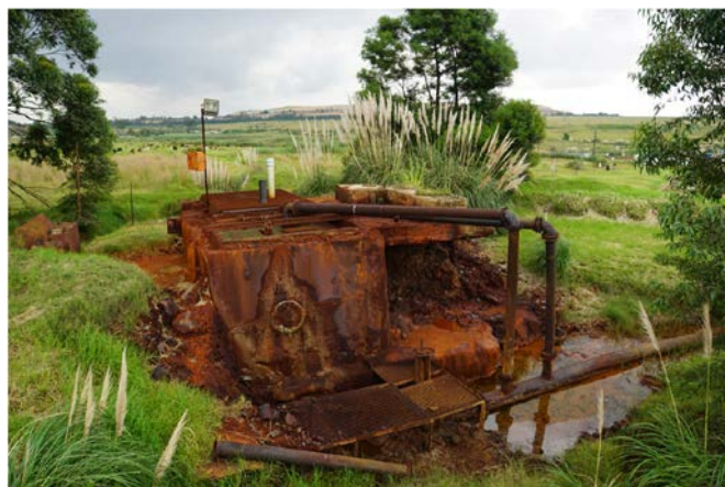
The Tweeloopiesspruit decant point in the Witwatersrand Western Basin in February 2017. Here the 'yellowboy' precipitate is a darker orange-brown colour.
